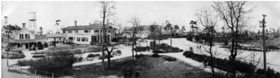
THIS 1903 VIEW FROM THE DEPARTMENT STORE BUILDING ILLUSTRATES THE PROPOSED 'VILLAGE POINT' TRIANGLE ISLAND
