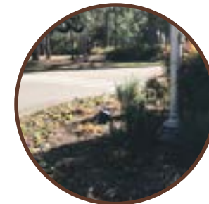
FLAG POLE LIGHT This light illuminates the flag pole in the center of downtown Pinehurst.
